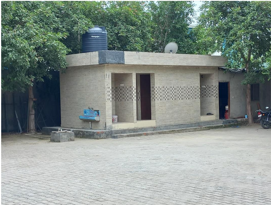
Photograph 5: The wash rooms / toilets within school and the water drinking tap ((Government school, village Wazidpur)
