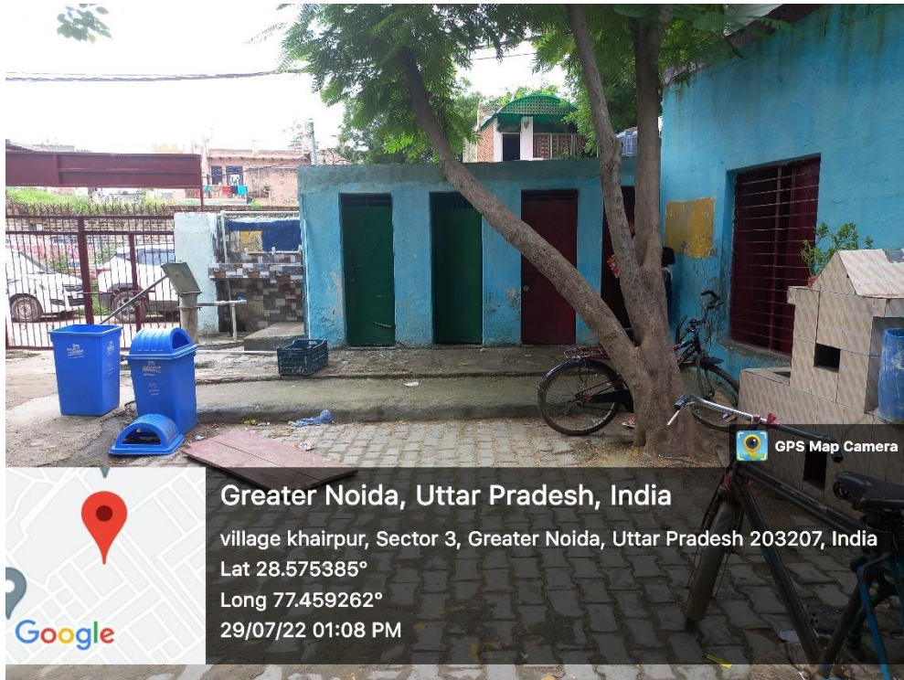
Photograph 3: The washroom and the handpump in the school premises (village Khairpur)
